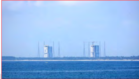
Two launch towers as seen from the sea (from the east). From left to right are the CZ-5 and the CZ-7 launch towers. Lightning towers are also visible in this picture. (credit: Chinese internet)
