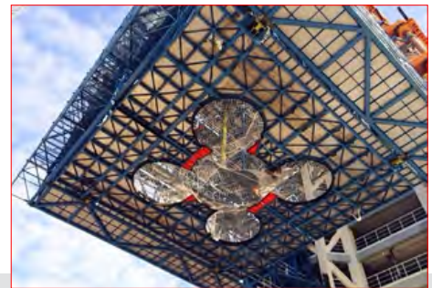
Close-up view of the bottom-most platform when closed, looking from the ground. The space for the 5 m diameter core stage and four strap-on boosters are seen at the centre of the platform. (credit: Chinese internet)
