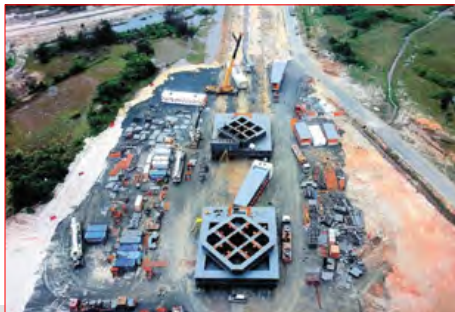
Two mobile transportation and launch platforms, one for CZ-5 and another for CZ-7, in assembly. Note the two "short sticks" near the platforms, which are the 58 m tall umbilical towers to be installed on the platforms. (credit: Chinese Space News/weibo)
