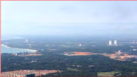
Full view of the Wenchang Space Launch Centre looking from the northeast. At the far left, near the sea coast, there are two launch towers - the front one is for CZ-7 while the back one is for CZ-5. At the far right are two vertical assembly buildings (VAB). (credit: Chinese internet)
