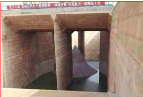
Flame diversion trough of the CZ-5 launch pad. (credit: Chinese internet)
