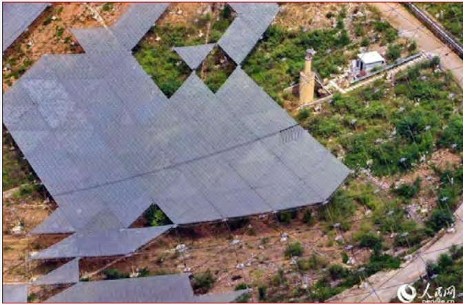
The panels of the FAST are partially installed. (credit: People's Daily)
