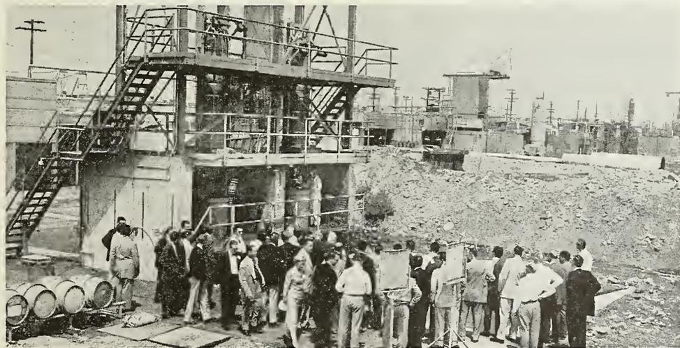
Newly-constructed test stand at Aerojet's Sacramento plant is shown in final stages of completion. This structure has been activated and is presently being used for full-scale static test firings of the complete second-stage system. Aerojet's Azusa and Sacramento test facilities are both being utilized for VANGUARD component and system evaluation and are currently in full operation.
