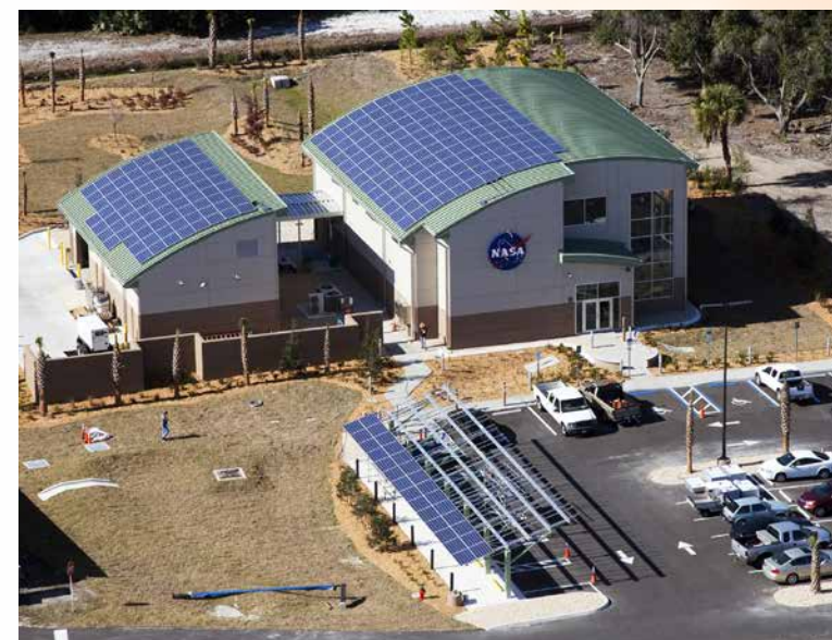
The Propellants North Administrative and Maintenance Facility at Kennedy Space Center produces an estimated 150 megawatt hours per year through an 80-kilowatt solar array. The system integrates two photovoltaic (PV) roof systems and a PV-covered electric vehicle charging canopy in the facility's parking lot. Photo credit: NASA/Frank Michaux
