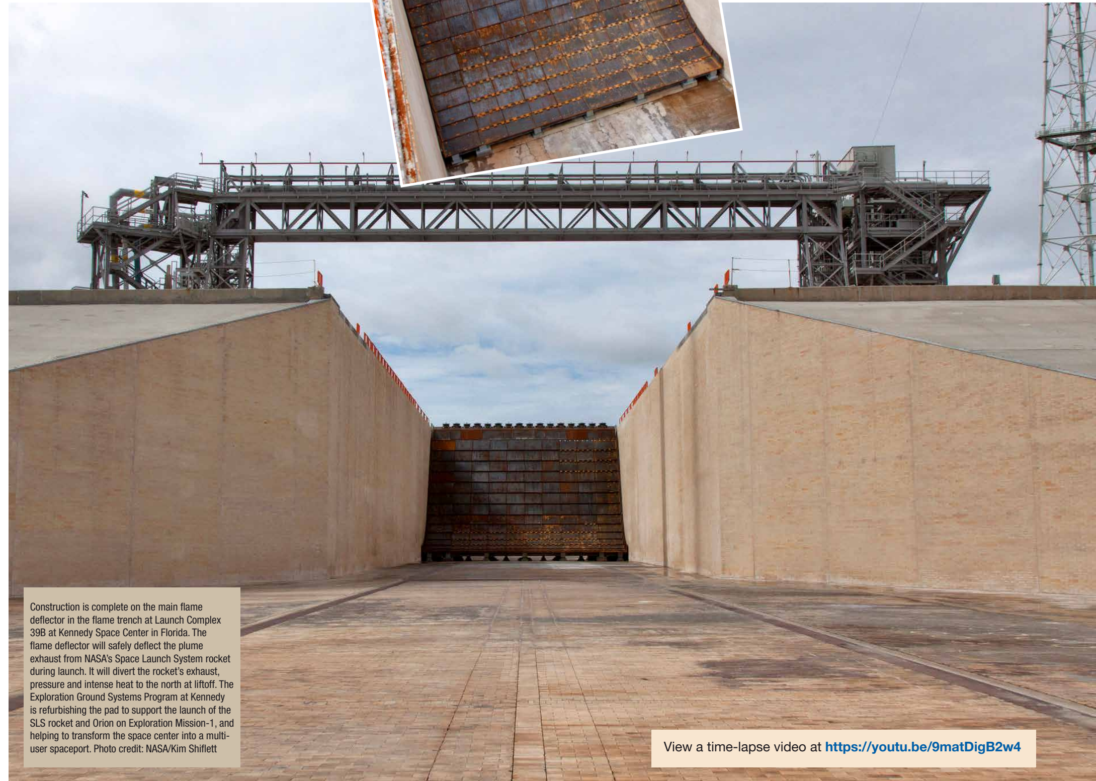
A close-up view of the main flame deflector in the flame trench at Launch Complex 39B at Kennedy Space Center in Florida. Photo credit: NASA/Kim Shiflett
