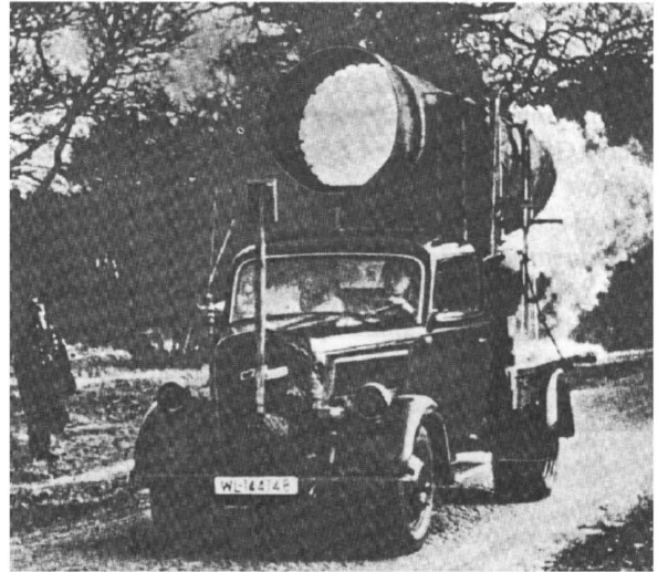
Fig. 7. Testing the ramjet's combustion space on the truck.
