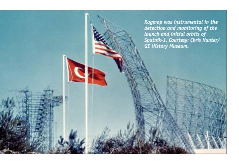
itored and recorded data from 13 Soviet rocket launches from the Kaputsin Yar test center. While the radar was originally intended to be a 'line of sight' detection system, atmospheric conditions during the summer and early autumn over south central Asia allowed the detection of missile launches well beyond the horizon, via atmospheric 'ducting,' which allows radio fre-
