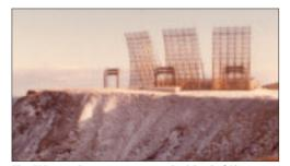
The FPS-17 radar system rests on the island of Shemya, Alaska. This version of the radar was used to detect the final phase of missile tests launched from Tyuratam. With several added antenna elements, this version of the FPS-17 covered four times the area covered by the system installed at Diyarbakir, Turkey. Courtesy James Moss.
