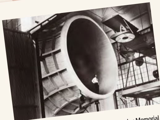
1927 Elton W. Miller, chief of aerodynamics at Langley Memorial Aeronautical Laboratory, stands in the Propeller Research Tunnel during studies on a Sperry M-1 Messenger, the first full-scale plane tested in the tunnel.
