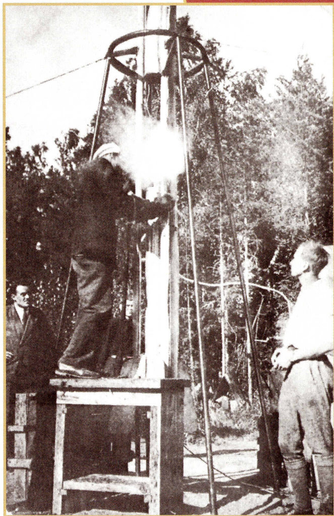
Korolev (far left) watches as a rocket club member fills the O9 rocket's oxidizer tank. Fueled by liquid oxygen and jellied gasoline, the O9 (below) was launched more than seven years after Robert Goddard's first liquid-fueled rocket.
