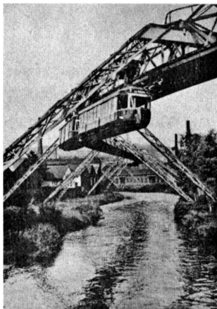
Two-car train of the Wuppertal Monorail traveling over the Wupper River
