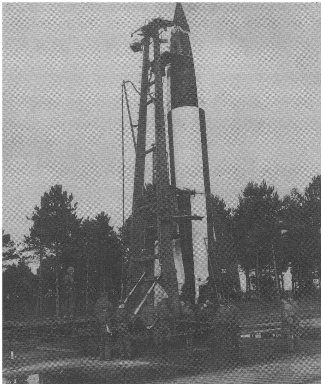
Figure 3 Electrical checkout of V2 prior to launch attempt on 1 October 1945, Cuxhaven.
