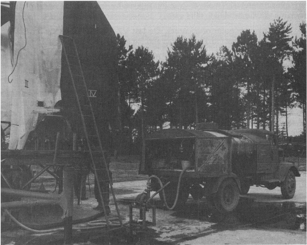
Figure 4 Loading hydrogen peroxide from tanker into V2 at Cuxhaven, 1 October 1945.
