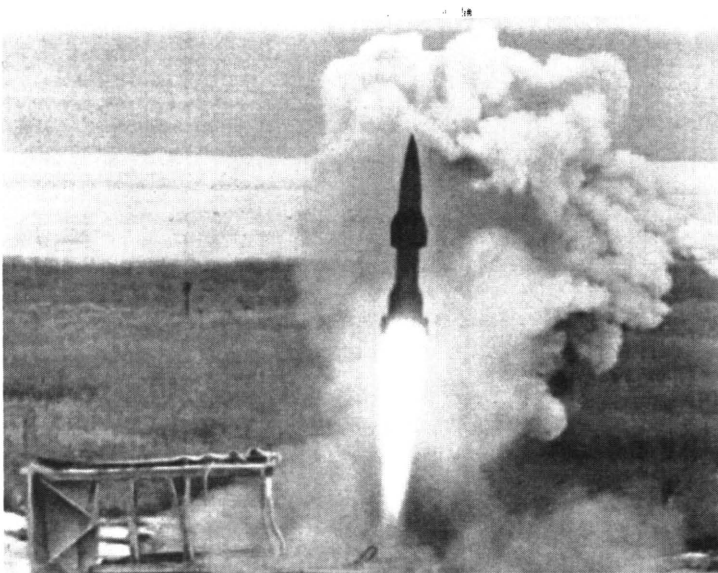
Figure 11–8: A test of the anti-aircraft missile, Wasserfall, on 23 September 1944. Credit: Bundesarchiv.
