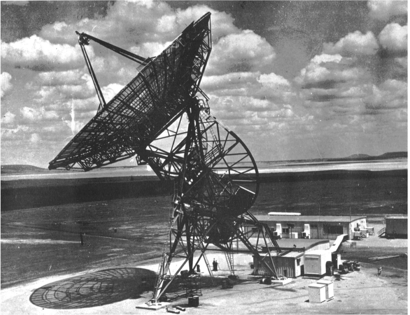
The 85-foot diameter antenna at Woomera, Australia, one of three that tracked and communicated with Mariner II. Others are located near Johannesburg, Republic of South Africa, and at Goldstone, California.
