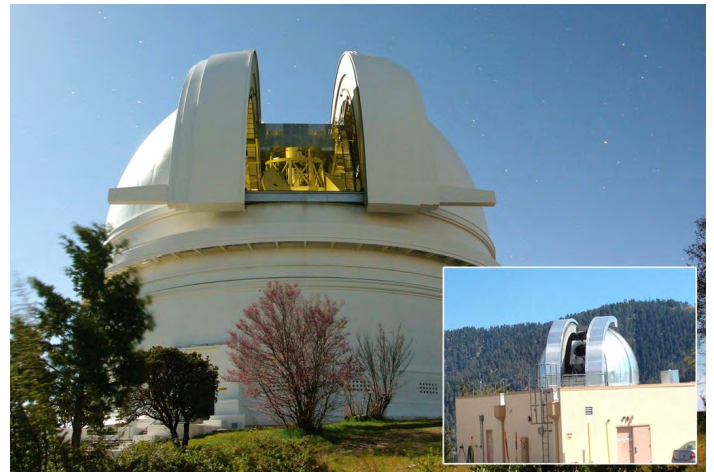
The 200-inch (5.1-meter) Hale Telescope at Caltech's Palomar Observatory in San Diego County will receive high-rate data from the DSOC flight laser transceiver and (inset) the ground-based laser transmitter at JPL's Table Mountain will send low-rate data to the flight transceiver. Image credit: NASA/JPL-Caltech/Palomar Observatory
