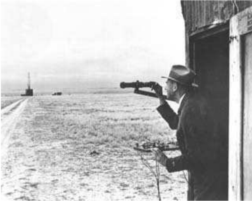
Figure 3.2: Robert H. Goddard tests a liquid-propellant rocket at his isolated research station outside Roswell, New Mexico, in the 1930s. The launch pad and support structure for the rocket are visible on the left, at the end of the dirt road. Goddard stands in the door of his “control room,” observing through a telescope with his left hand on the launch controls. Courtesy of NASA Headquarters, image number 74H-1245.
