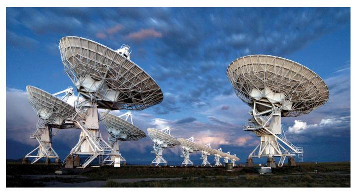
▲ SPLITTING THE FEED The Very Large Array is a collection of 27 radio antennas in Socorro, New Mexico. Each antenna in the array measures 25 meters (82 feet) in diameter and weighs about 230 tons. In the COSMIC SETI initiative, feed splitters will copy the data that the VLA collects, enabling special correlators to analyze astronomical data for extraterrestrial intelligence.
