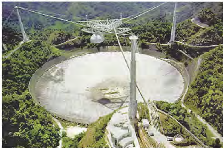
So far, Project SERENDIP has gathered an impressive amount of data using the Arecibo radio telescope in Puerto Rico. The telescope's huge dish covers an area of about 50 hectares (20 acres). Photo: David Parker/Science Photo Library, courtesy of the NAIC Arecibo Observatory, a facility of the NSF
